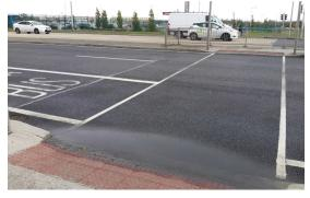
Figure 3.5 Ponding at existing crossing
